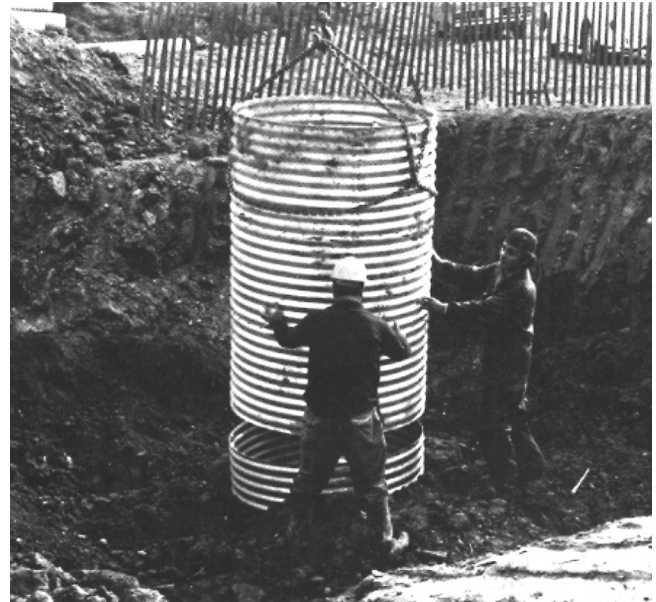
Placing Riser Section on Pipe Stub.
