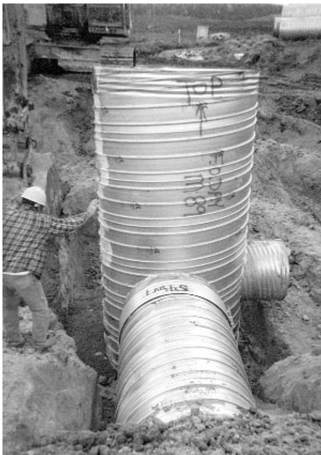
In-Line, Shaft-Type Manhole.
