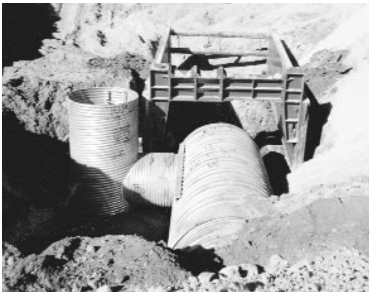
Offset, Shaft-Type Manhole on a Slab.
